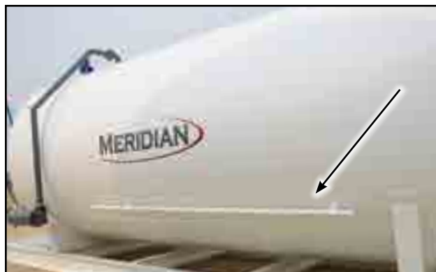
Fig 20 - Dip stick location
