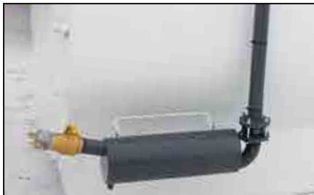
Fig 17 - Bottom fill tube with cam lock
